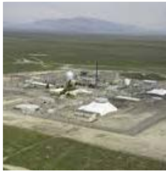
Transfer of Np stored at INL to ORNL
